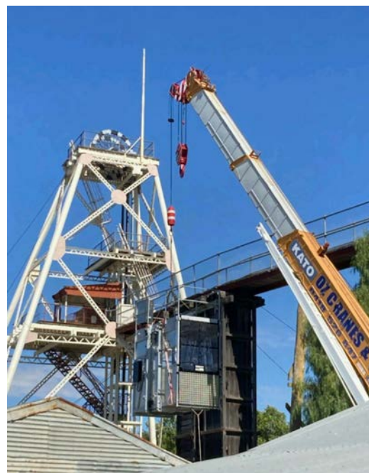
New Alimak lift installation.
